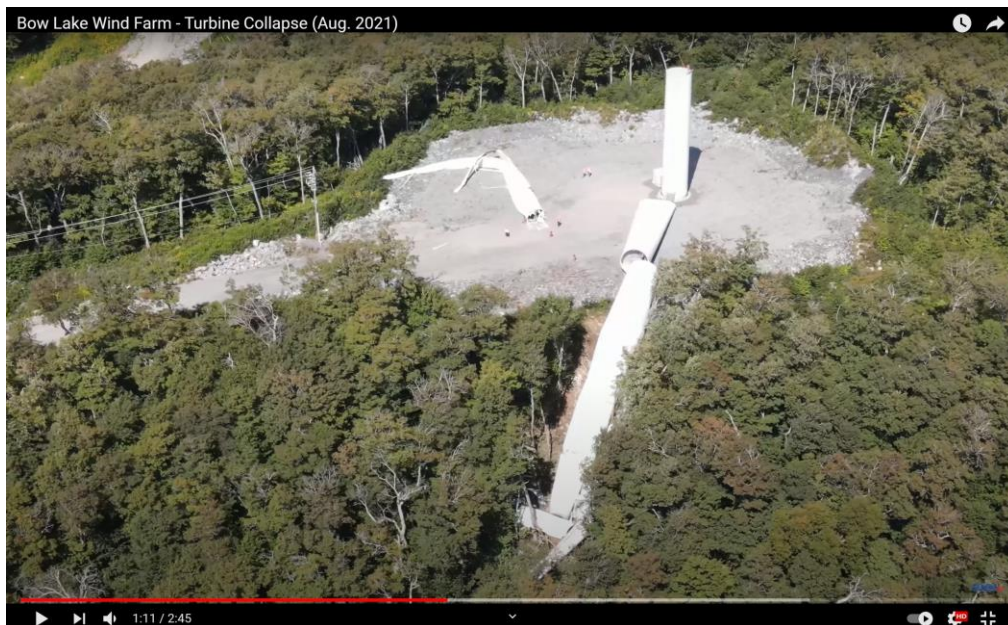
Collapse of Bow Lake wind power facility near Sault Ste. Marie. Click on image to see video.
